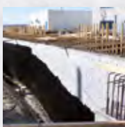
External basement waterproofing
